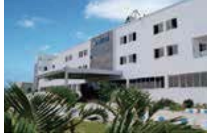
Rudrapur Plant (Green Building)
